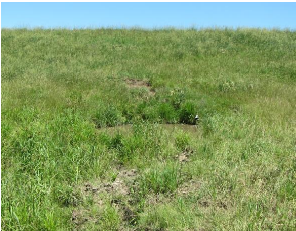
Pond 205 standing below and facing the dam.
