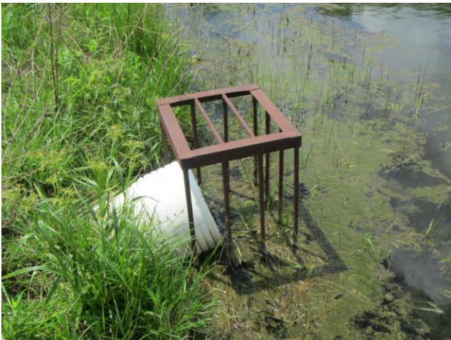
Pond 183 stand pipe. This also shows that the pond retention area was full, but water did not overflow into the terrestrial vegetation.
