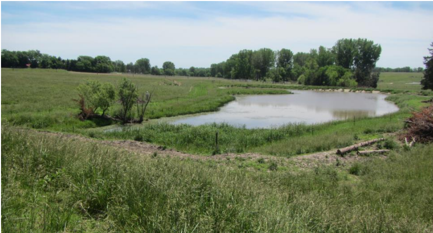
View of the downstream area as photographed from the dam of pond 230 which had no stand pipe.
