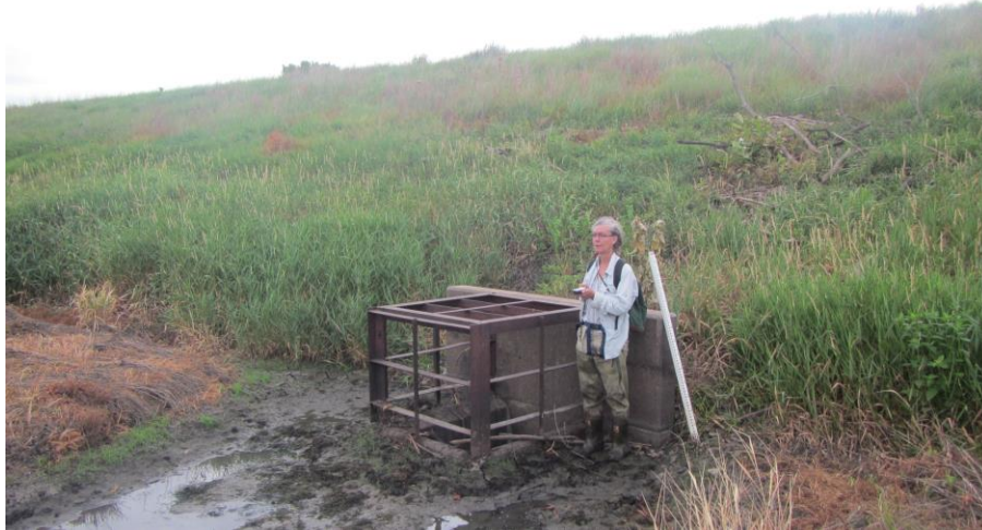
Figure 15. Standing at the pond-side base of a large dam (high point elevation 6.2 m above water level, 1.99 m above spillway low point) which is the watershed dam of pond 268.
