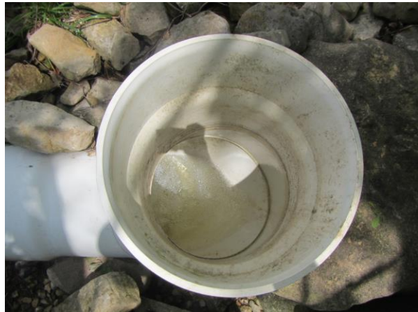
Pond 183 with view (right) inside the pipe showing water that leaks out of a joint in the pipe.
